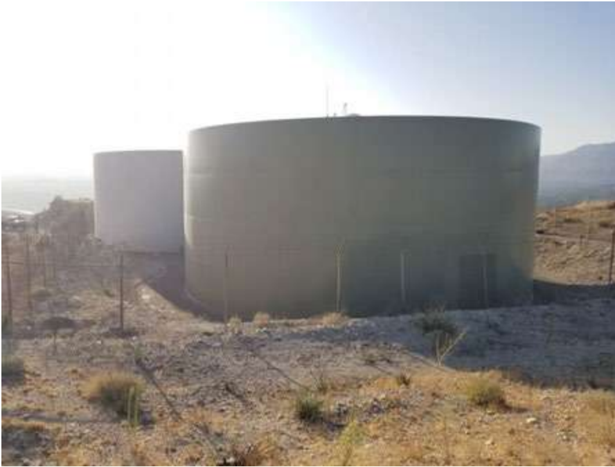
Photo 1: Existing Tanks to Remain (View SE)
