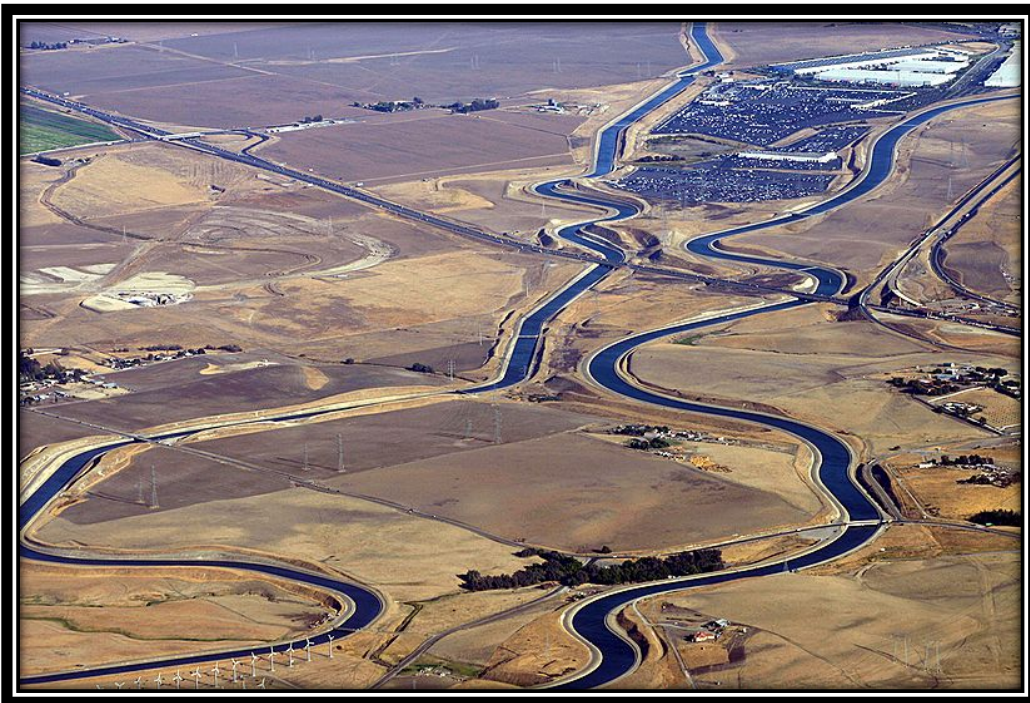
Aerial photo of the California Aqueduct at the Interstate 205 crossing. Photo courtesy of Wikipedia.com
