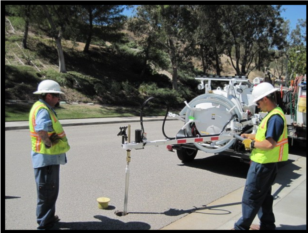
Daniel Liles, Utility Worker I, and Jon Mahar, Utility Worker II, exercising a valve with a new, remote controlled valve exercising machine. The new machine maintains a consistent torque and monitors the number of turns to close a valve, thus reducing valve breakage.
