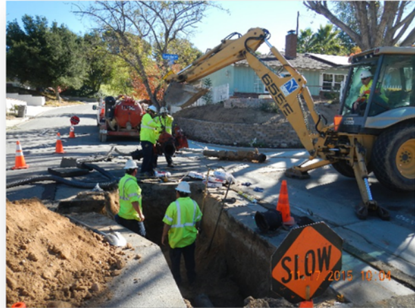
Pipeline Replacement - Shadeland
