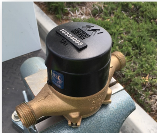
Meter Replacement – Master Meter
