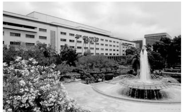
Los Angeles County Hall of Administration
