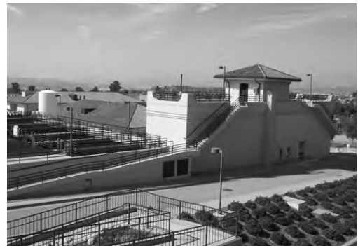
Rio Vista Water Treatment Plant
