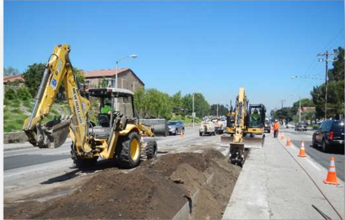
Pipeline Replacement - Newhall Avenue
