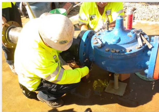
Large Meter Replacement - Castaic
