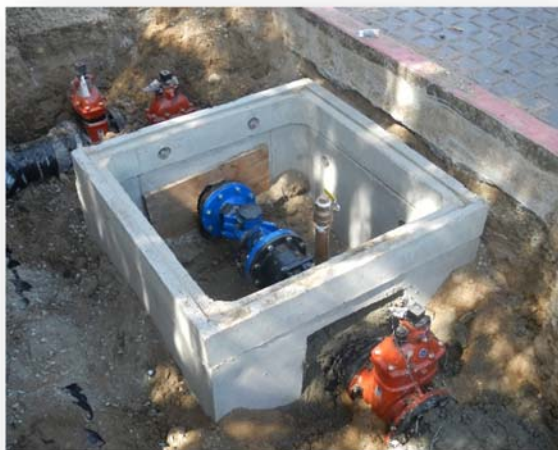
Large Meter Replacement - Valle del Oro
